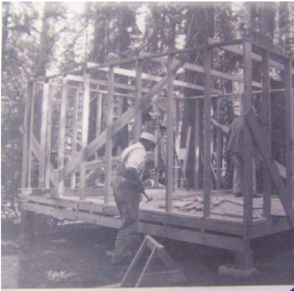
Building the "Madras" cabin
