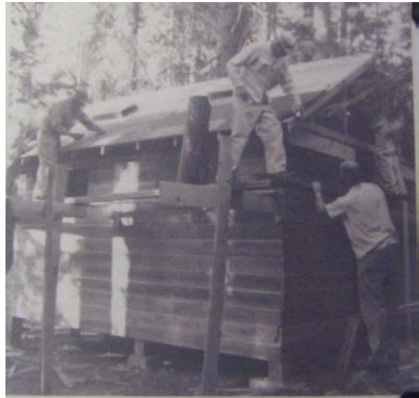
Building the "Madras" cabin
