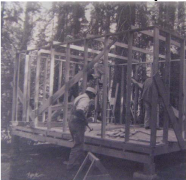
Building the "Madras Cabin"
